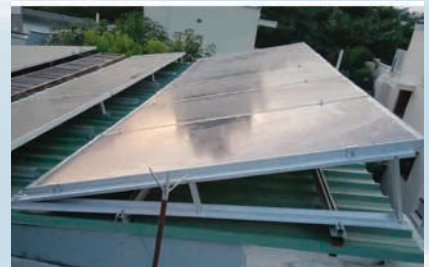
Metal Roof - North Tilt
