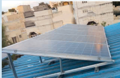
Metal Roof - South Tilt
