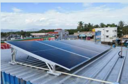
Metal Roof - East West
