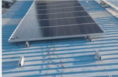
Metal Roof South
